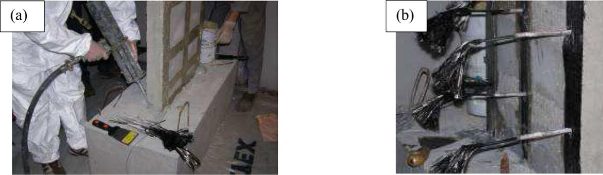
Figure. A-4: (a) Injecting resin into the anchors; (b) Implementation of anti-buckling anchors
