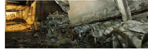
GOTHARD tunnel, FAURE & HEMOND
